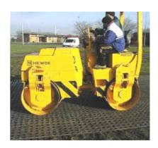
After about 3-4 rows are laid out, they should be rolled in leaving the last row unrolled.
